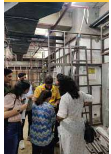
Discussion on-site to solve metal junctions
